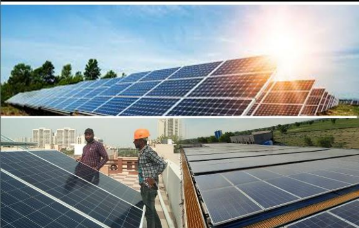
SOLAR POWER PLANT INSTALLATION
